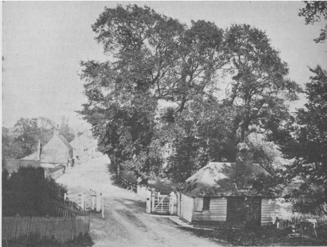
Bramber Tollgate, demolished in 1885
